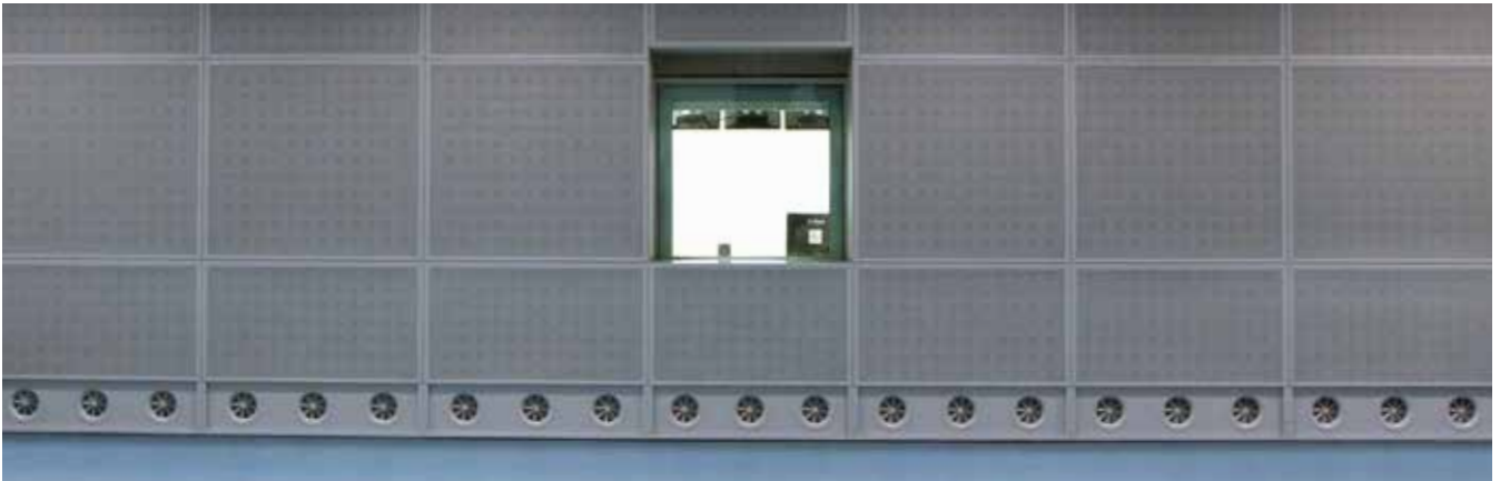
Indoor shooting range, Düsseldorf, Germany Guaranteed protection of the shooter against harmful gases and respirable dusts
