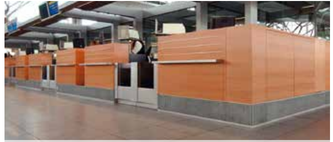
Plinth diffuser integrated in the front of counters. Front face built of shock proof stainless steel LSE material. Stuttgart Airport, Terminal 3, Germany
