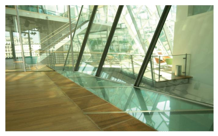
Wooden displacement floor diffusers. Front face 23mm plywood with oak veneer on 30mm high steel grid, mounted in stainless steel frame.
