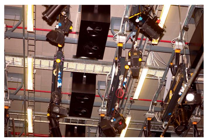
Tailor made duplex variable air pattern swirl diffuser with displacement section. Designed for 2 airflows with same sound power level and pressure loss.
