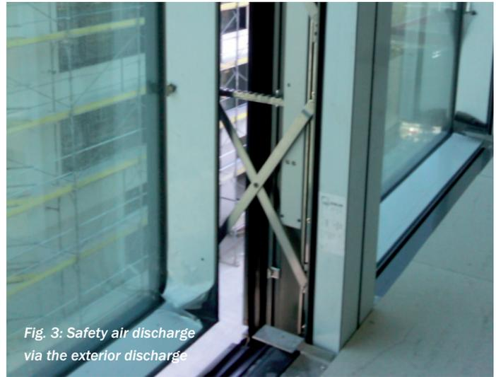
Fig. 3: Safety air discharge via the exterior discharge
